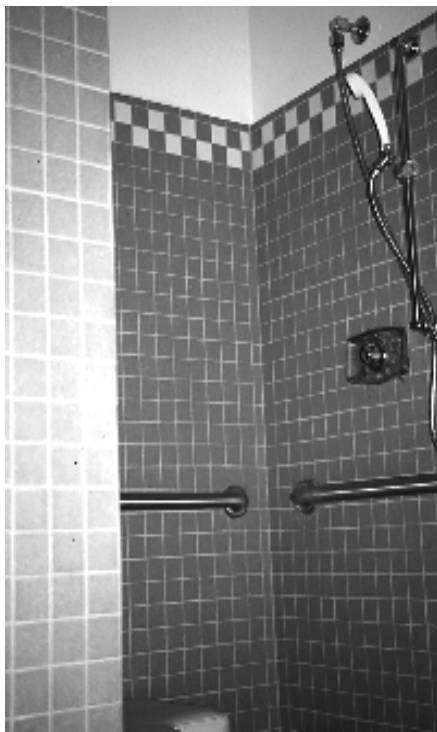
This shower which allows wheelchair access is located in the Florida Department of Environmental Protection as part of the Bicycle/Pedestrian Commuter Center located there.
